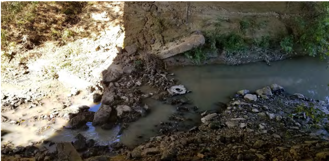
Figure 2. Johnson Creek at Austin Road Bridge showing minimal riprap protection under the bridge.
