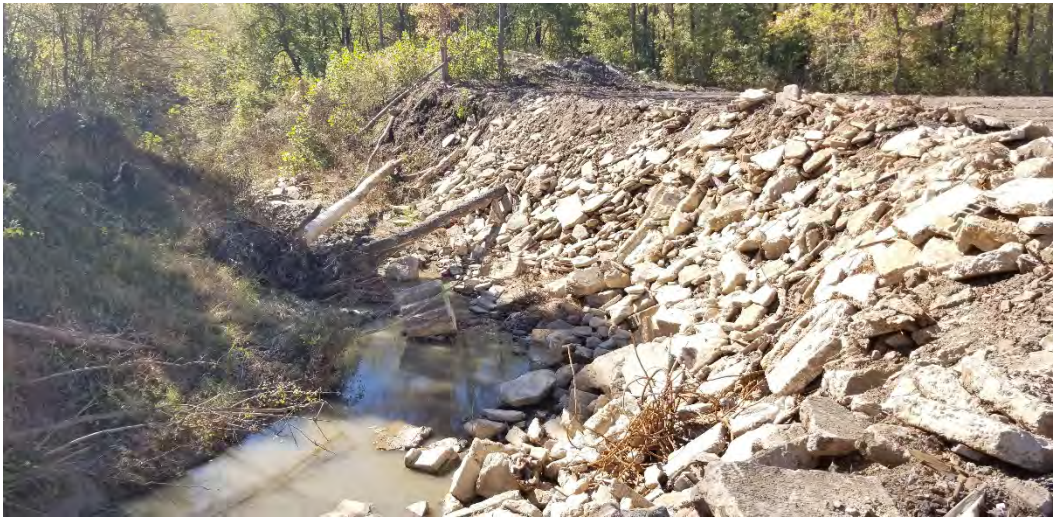
Figure 23. Johnson Creek Reach 2: Concrete bank revetment at Odums Crossings Subdivision
