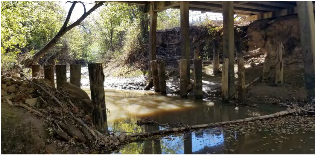
Figure 32. Johnson Creek Reach 3: Limited riprap and concrete bank revetment at the Austin Road Bridge.
