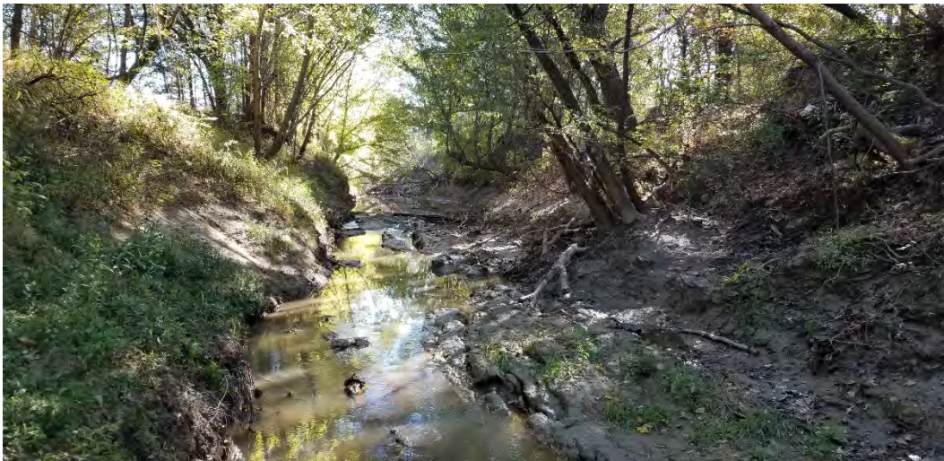
Figure 4. Johnson Creek-Baldwin Road Bridge-looking upstream at degrading channel, trees sliding in on right bank
